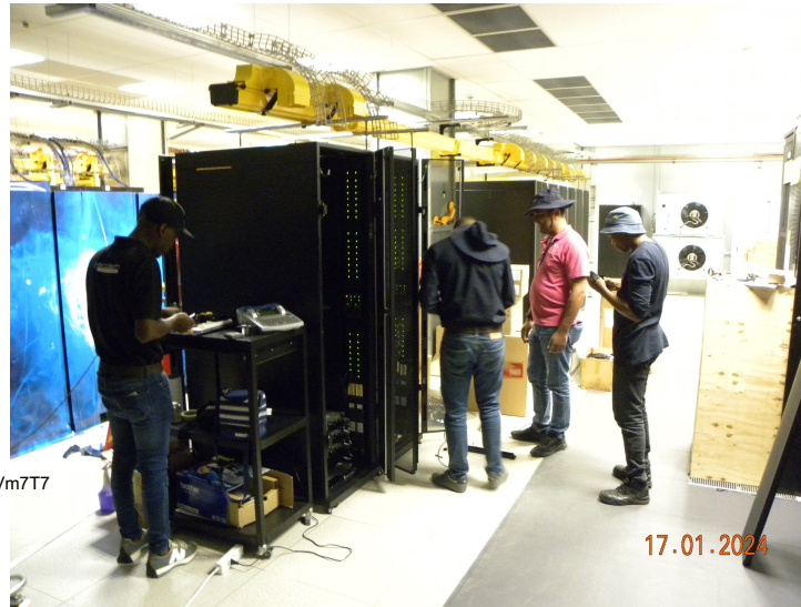
Above & Right: Successful installation & configuration of the AA0.5 servers in the Karoo Array Processor Building on site
