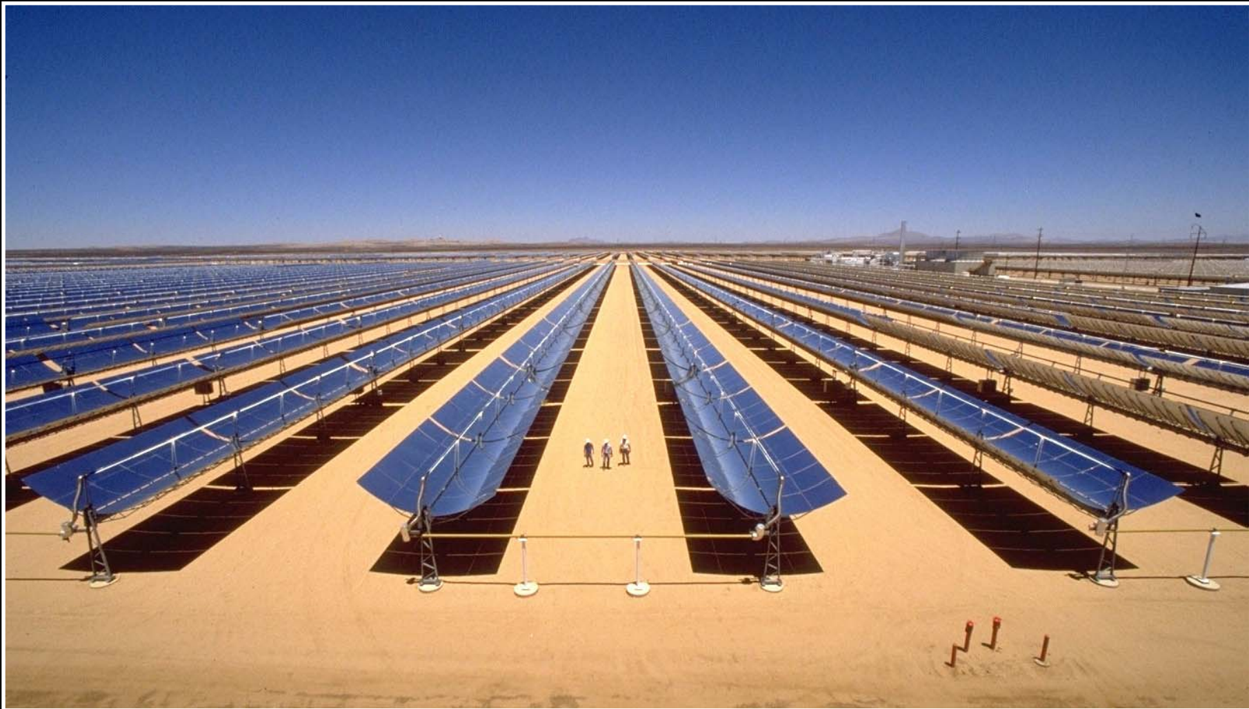
Parabolic trough CSP plant (150MW), Kramer Junction, California
