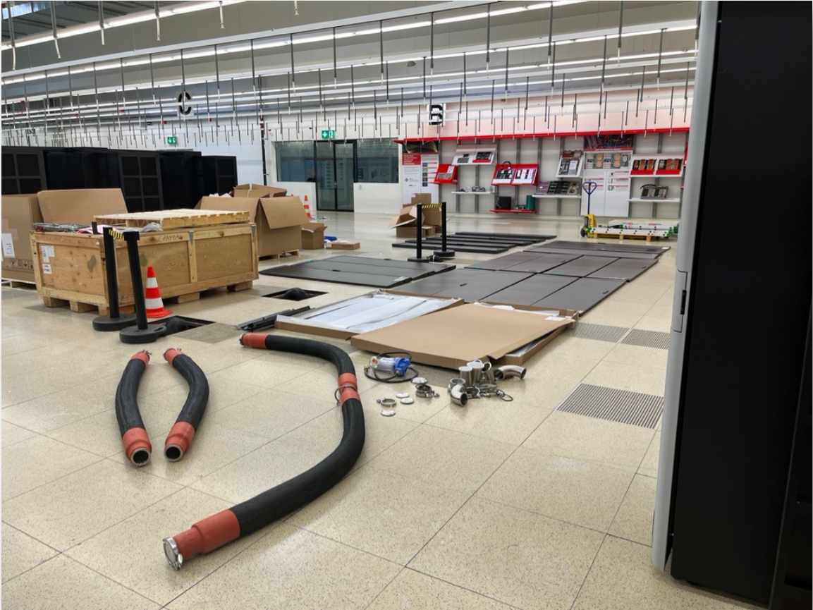
Internal pipes and doors and panels
