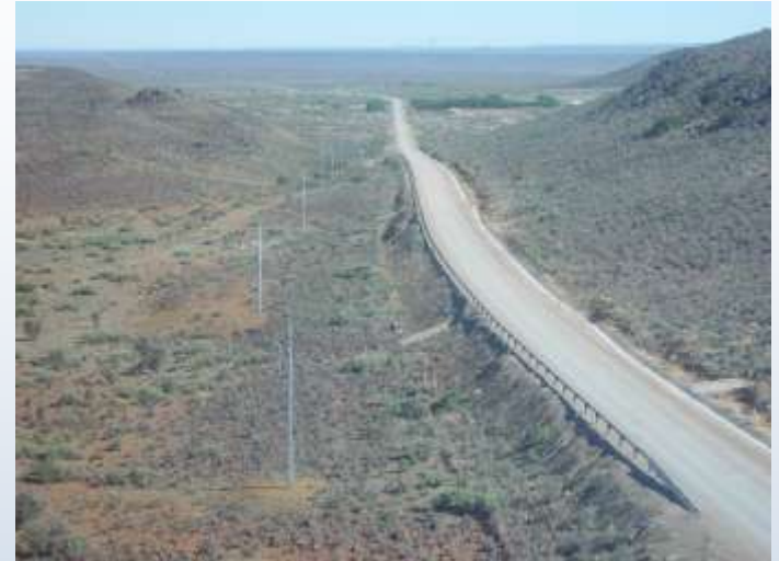
New 33 kV Powerline with MASS fibre optic cable approaching Core Site
