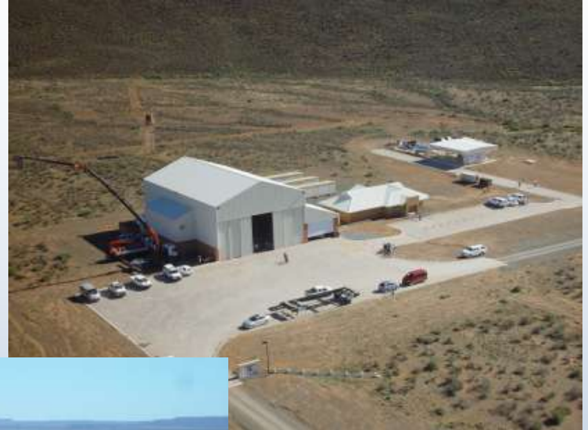
Core Site Complex
