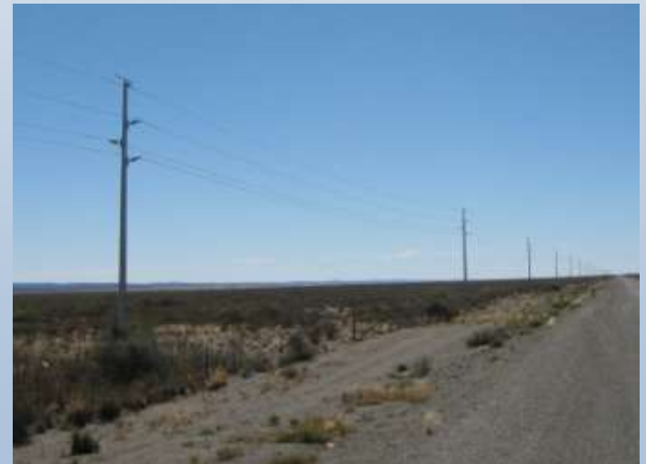
New 33 kV Powerline with MASS fibre optic cable approaching Core Site
