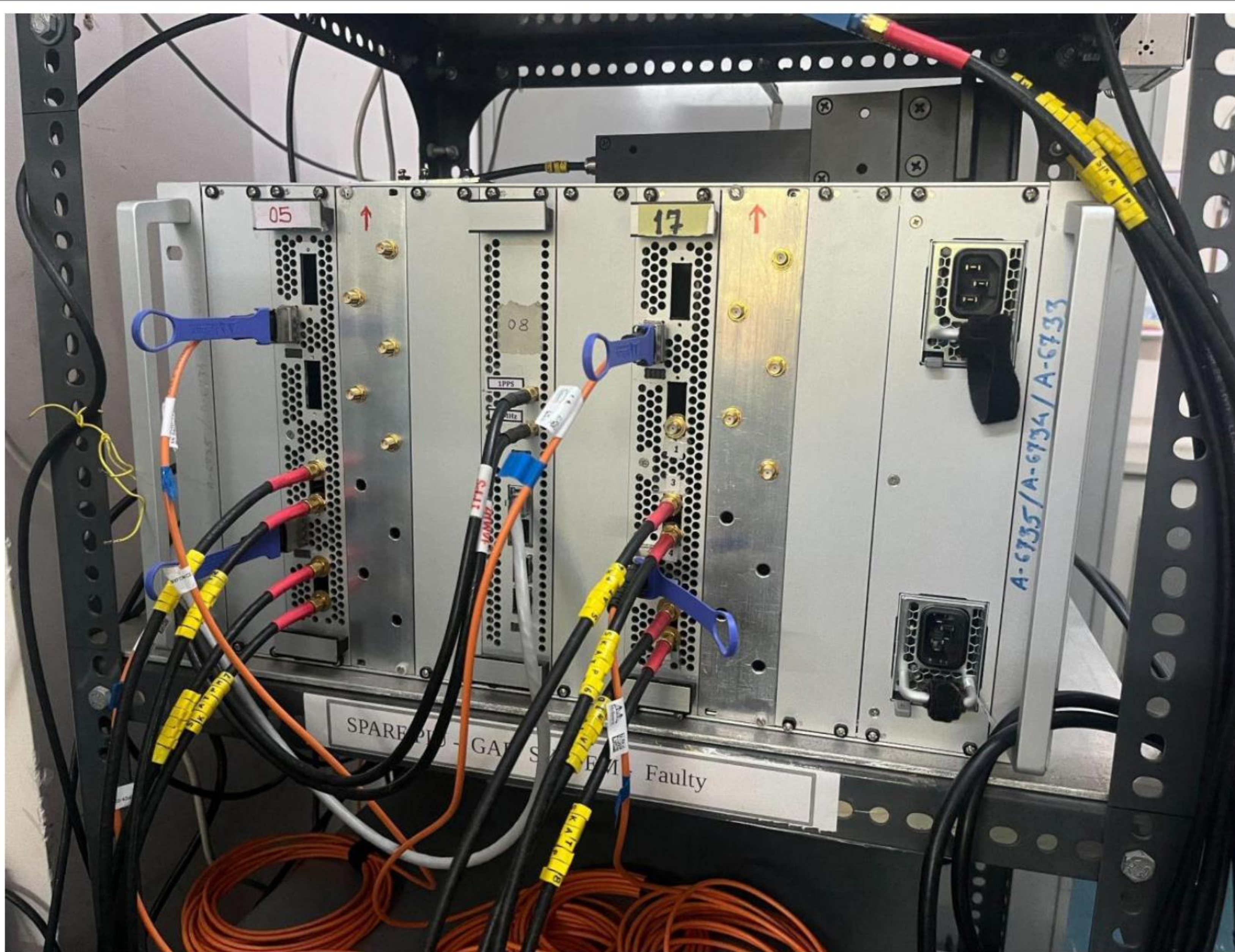
SPS - Sub rack delivered at GMRT in India
