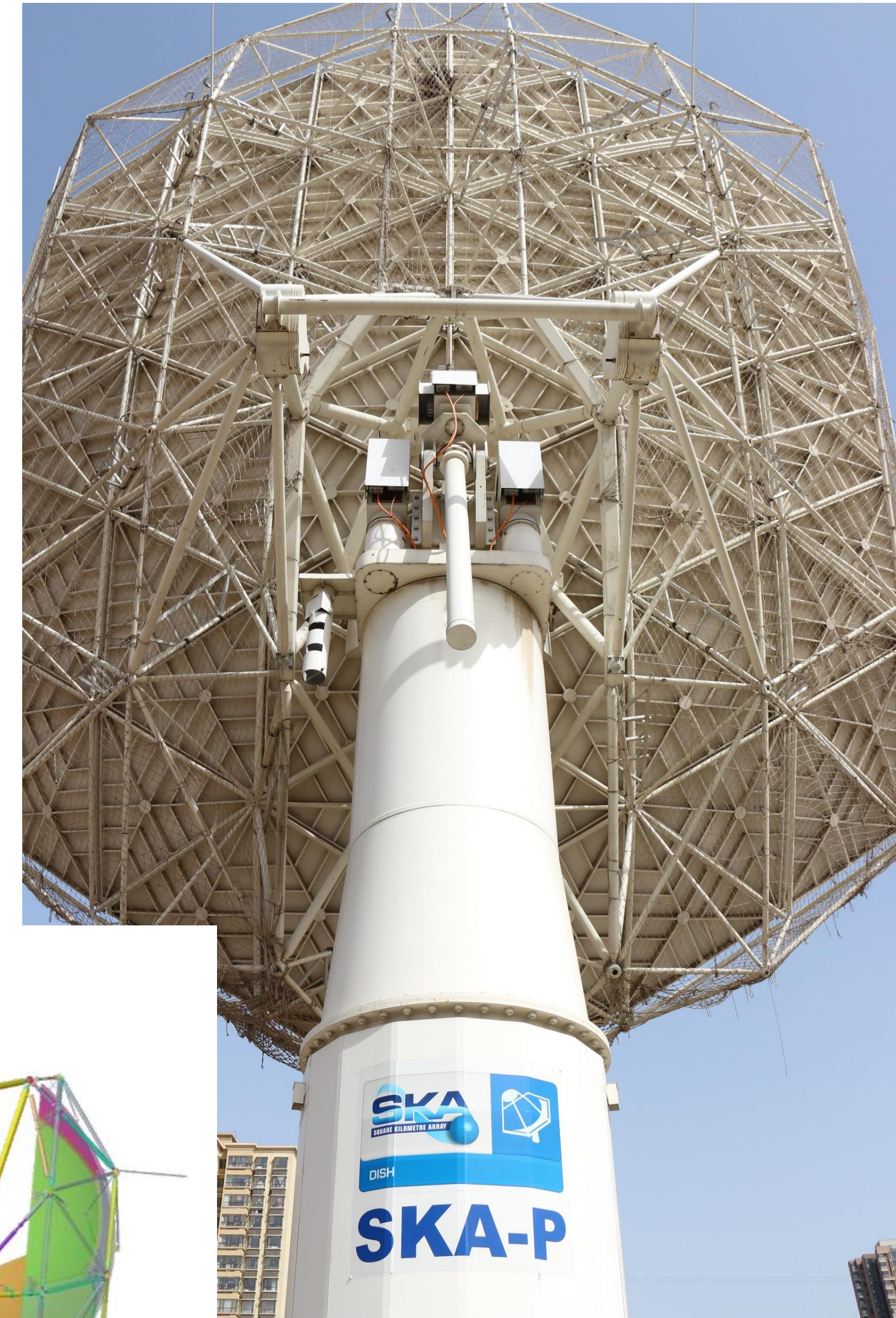
Main Reflector Backup Structure
