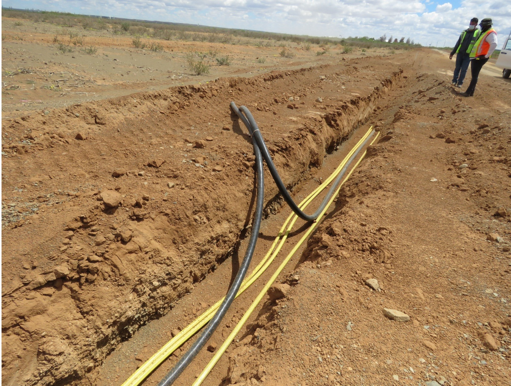
Fibre & Power trenching
